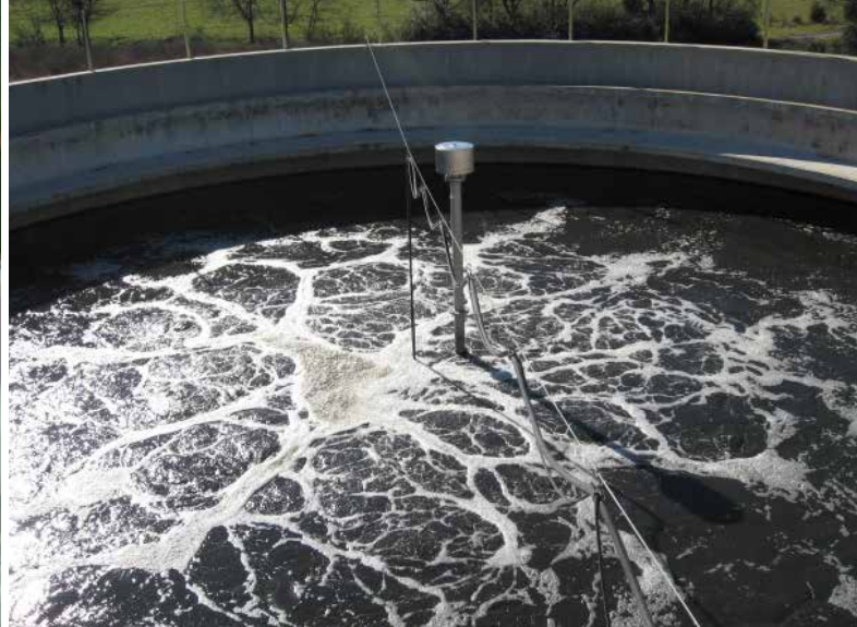
Installation in post aeration basin
