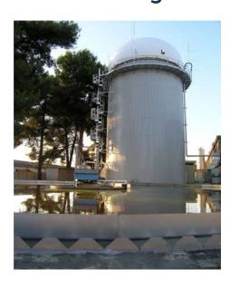
Digester in which a particular "granular" anaerobic sludge grows. Used directly on wastewater, as long as they have soluble COD (sugars, starches, etc.), with COD>2000 mg/L.
