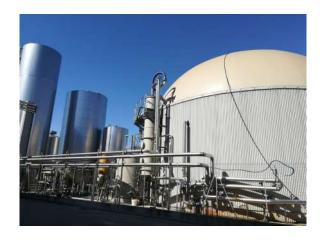
Complete mixed process with anaerobic biomass recirculation, which allows biomass concentration increase and a reduction of digester volume. Suitable for streams with COD > 40 000 mg/L.
