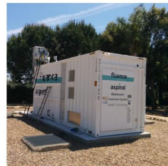
Figure 13. CENTA case study demonstrates that Fluence’s Aspiral MABR system meets EU regulatory requirements
