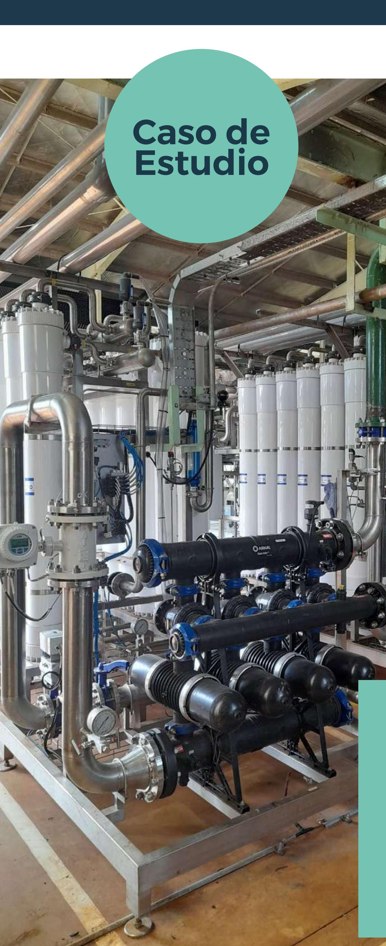
A photograph showing a complex industrial water treatment system. It features several large white cylindrical filter units, various pipes in different colors (blue, black, silver), and a network of valves and fittings. The equipment is mounted on a metal frame and is set against a background of a steel structure with visible beams and overhead piping.
