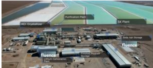
Lithium mine brine treatment, Argentina
