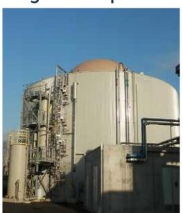
Biogas is rich in hydrogen sulphide, which is harmful to cogenerators and boilers. Unlike its competition, Fluence's biogas desulphurization systems do not involve air blowing into the digester dome or traditional scrubbing of the biogas with chemical reagents.
